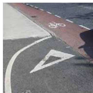
Abrupt transition to carriageway
